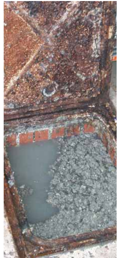
Blocked drains and sinks like can be the cause of many environmental and health issues and result in costly remedial works.
