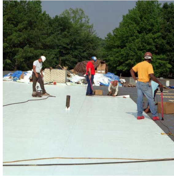
For cool roofs with reflective coatings, the roof should be cleaned at least once a year with a high-pressure water spray.
