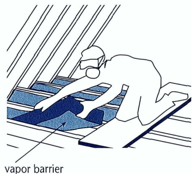
Figure 8: Begin laying insulation at the outer edge of the attic.
