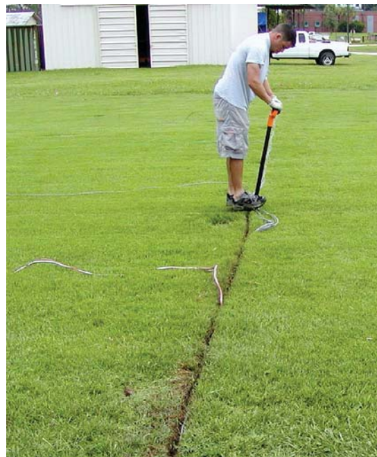
Figure 26. A conventional slit trench, which should only be used when placing wiring in conduit.
