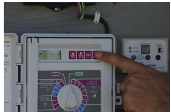
Figure 40. Manual start of irrigation timer while SMS controller is “On Hold” to test proper operation.
