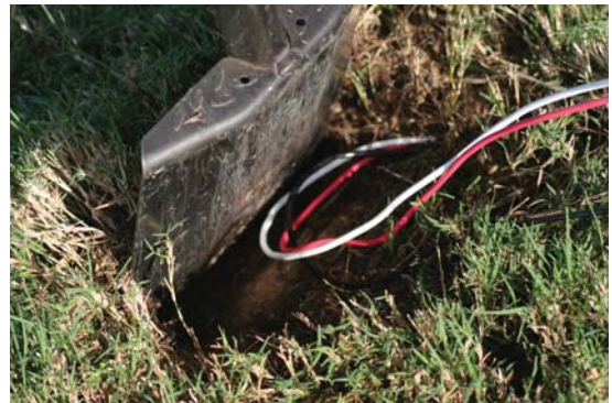
Figure 23. Lifting shovel within the lift trench to create room for SMS wiring.
