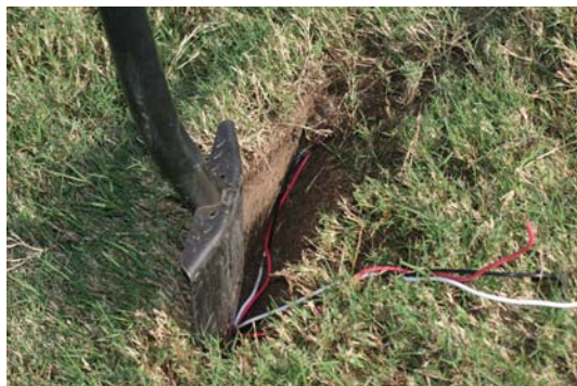
Figure 24. Placing sensor wires while continuing lift trench
