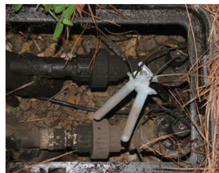
Figure 33. Enclose all wire nuts in direct burial connectors.
