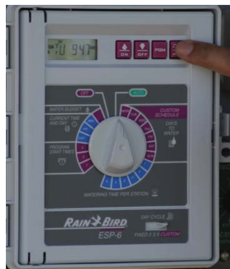
Figure 39. Manual start of the irrigation time clock to saturate area around SMS for calibration.
