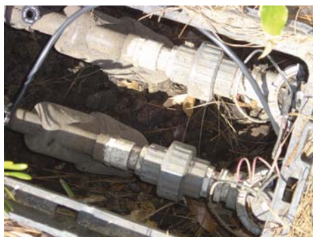
Figure 29. Uncover the irrigation zone valve box.
