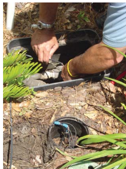
Figure 30. Disconnect the existing wiring connection between the irrigation timer and zone valve.
