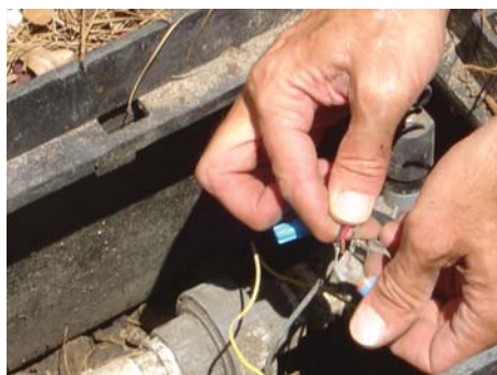
Figure 32. Connect the wires from the soil moisture sensor to the zone valve.
