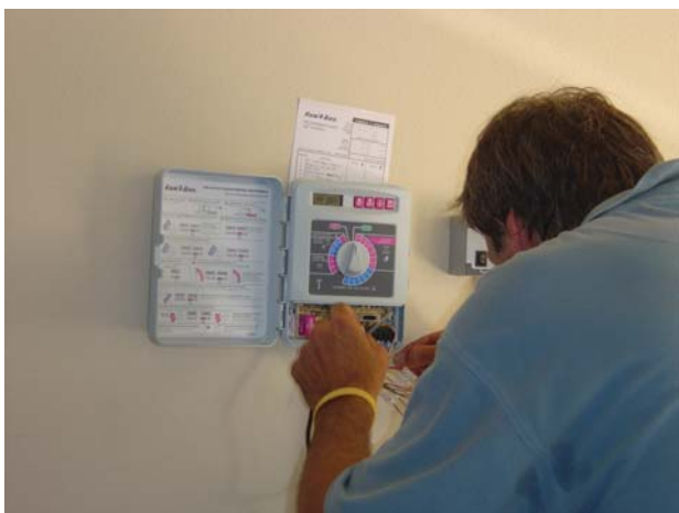
Figure 36. Connect SMS controller wiring to the irrigation timer wiring.
