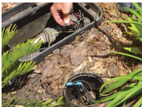
Figure 31. Prepare the soil moisture sensor and zone valve for connection.
