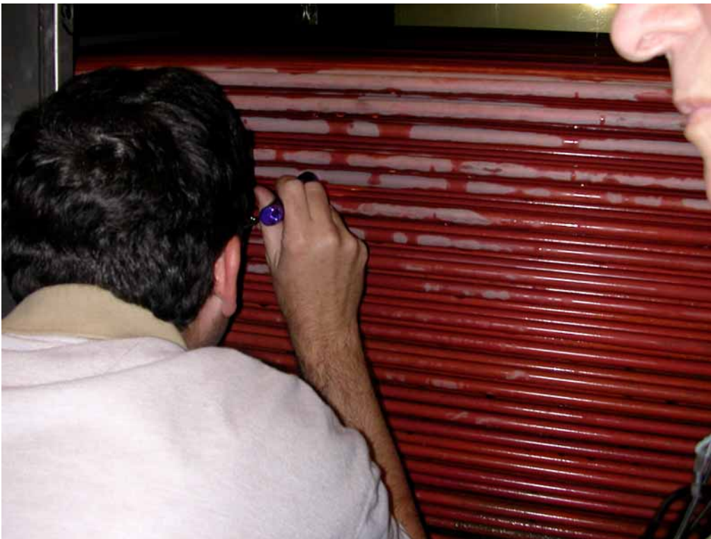
Figure 54: Mark Gentili, LADWP, inspecting Beverly tubes, May 2003
