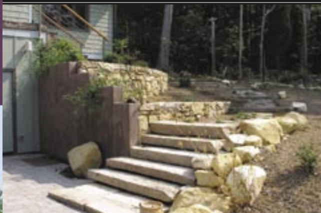
Steps are reclaimed Durham city curbs; terrace walls from site stones.
