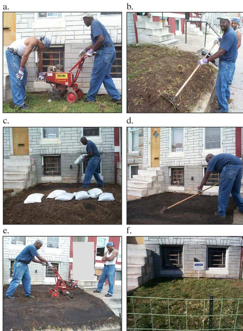
Fig. 1. Biosolids compost amendment process: (a) initial rototilling; (b) surface preparation; (c) biosolids compost application; (d) forming a 6–8 cm layer of biosolids compost; (e) rototilling to a depth of 20 cm; (f) emerging grass cover.
