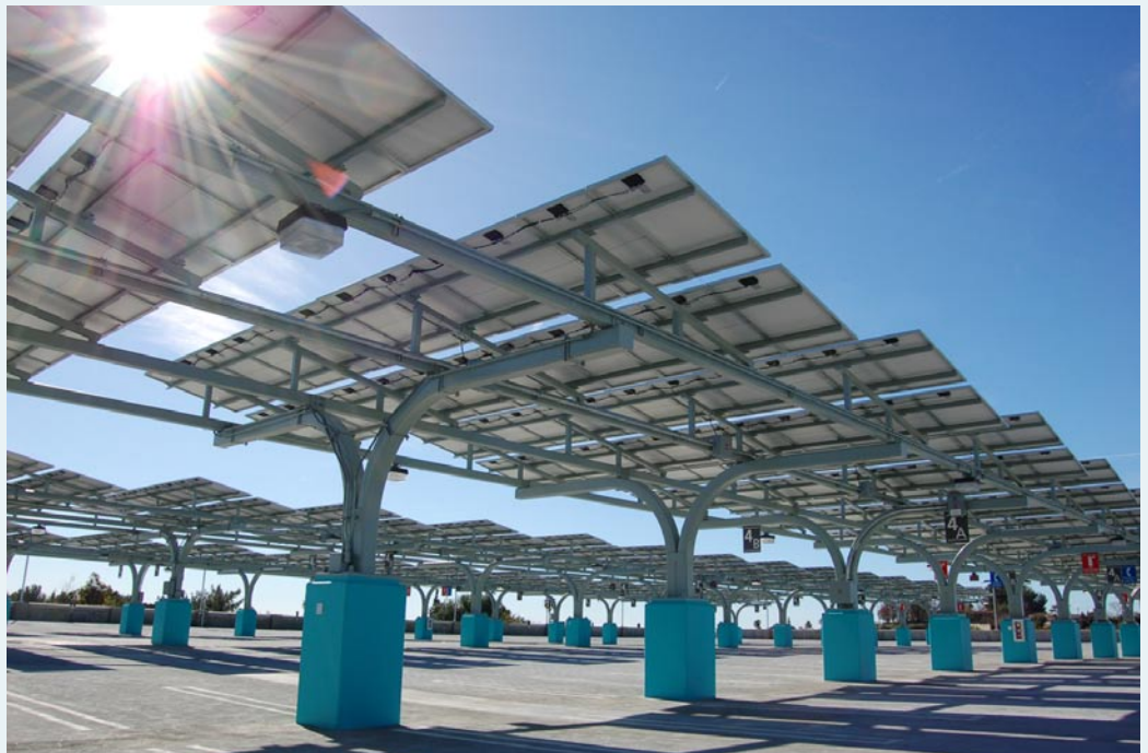
Solar (photovoltaic) panels are installed on a shade structure above a parking structure, Los Angeles Community College District
