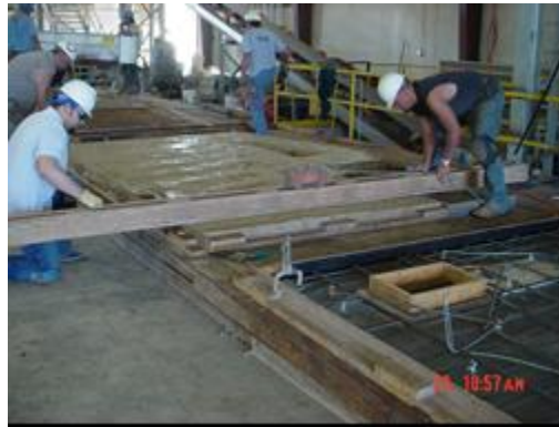
b) Placing Concrete
