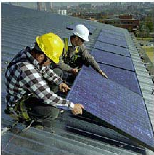
Workers install flat-plate PV panels on the Natatorium for the 1996 Summer Olympics in Atlanta.
