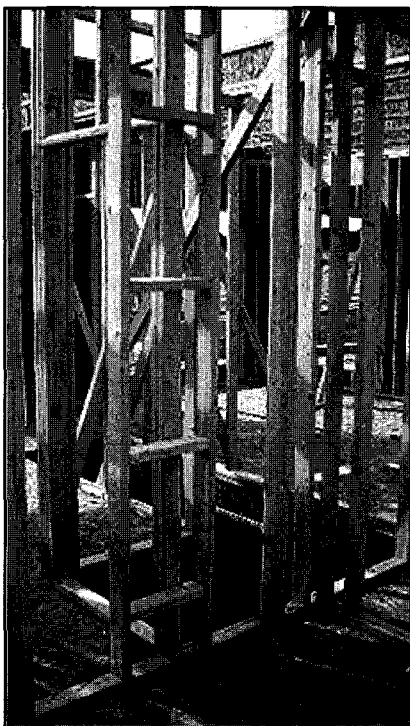
Ladder framing reduces the number of studs required to frame intersecting walls.
