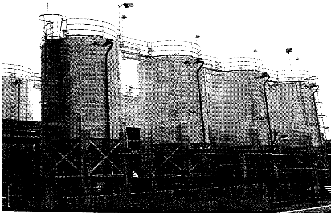
Figure 200.11 View One of a Solvent Recycling Plant
