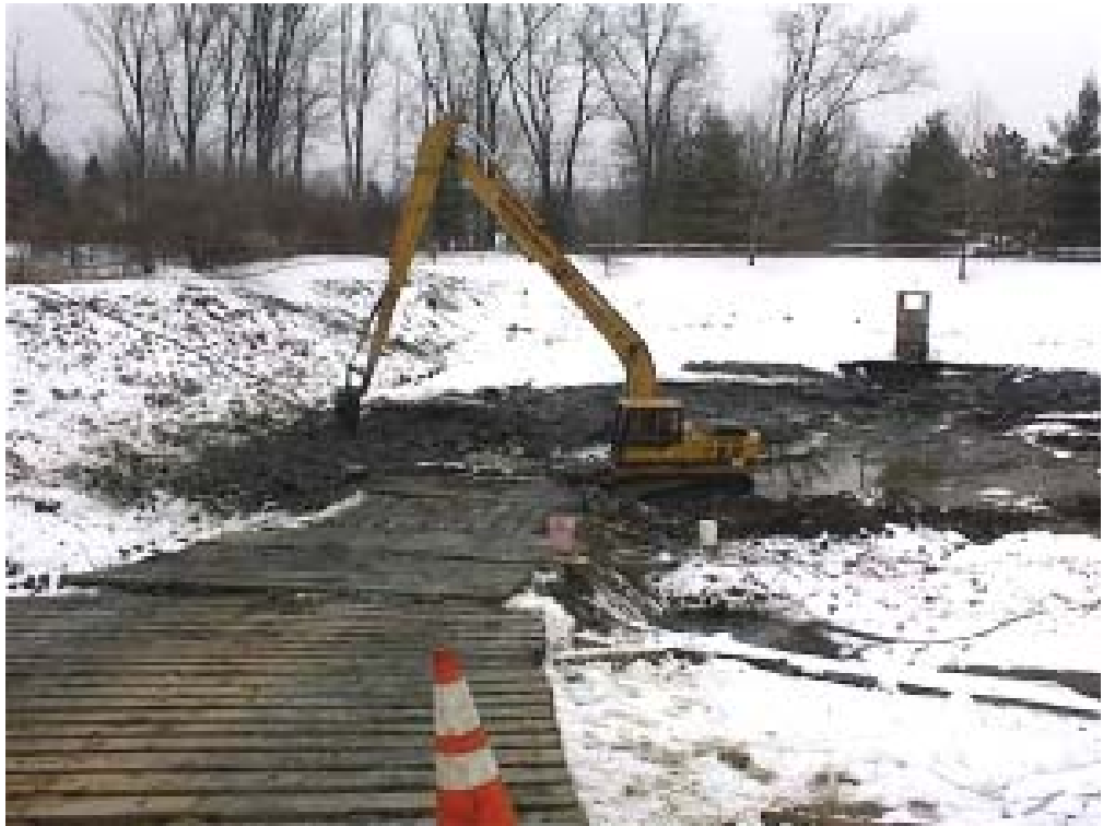
Fig. 9. Dredging following drawdown during winter at a development in Willistown Township (photograph courtesy of R. Stephanou).
