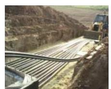
3. "Pigtail" pipes coming from the individual heat exchangers join at the valve pit (lower left).
