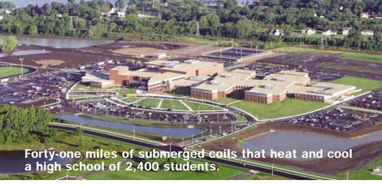
In the fall of 2001, Fond du Lac High School opened its doors to students and began operation of the largest geothermal pond system in the United States. Using energy from the earth, geothermal technology provides a reliable and economical heating and cooling alternative for schools and other large commercial institutions.
