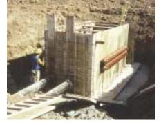
4. This box, called the valve pit, joins the heat exchanger pigtail pipes to the main feed lines for the school.
