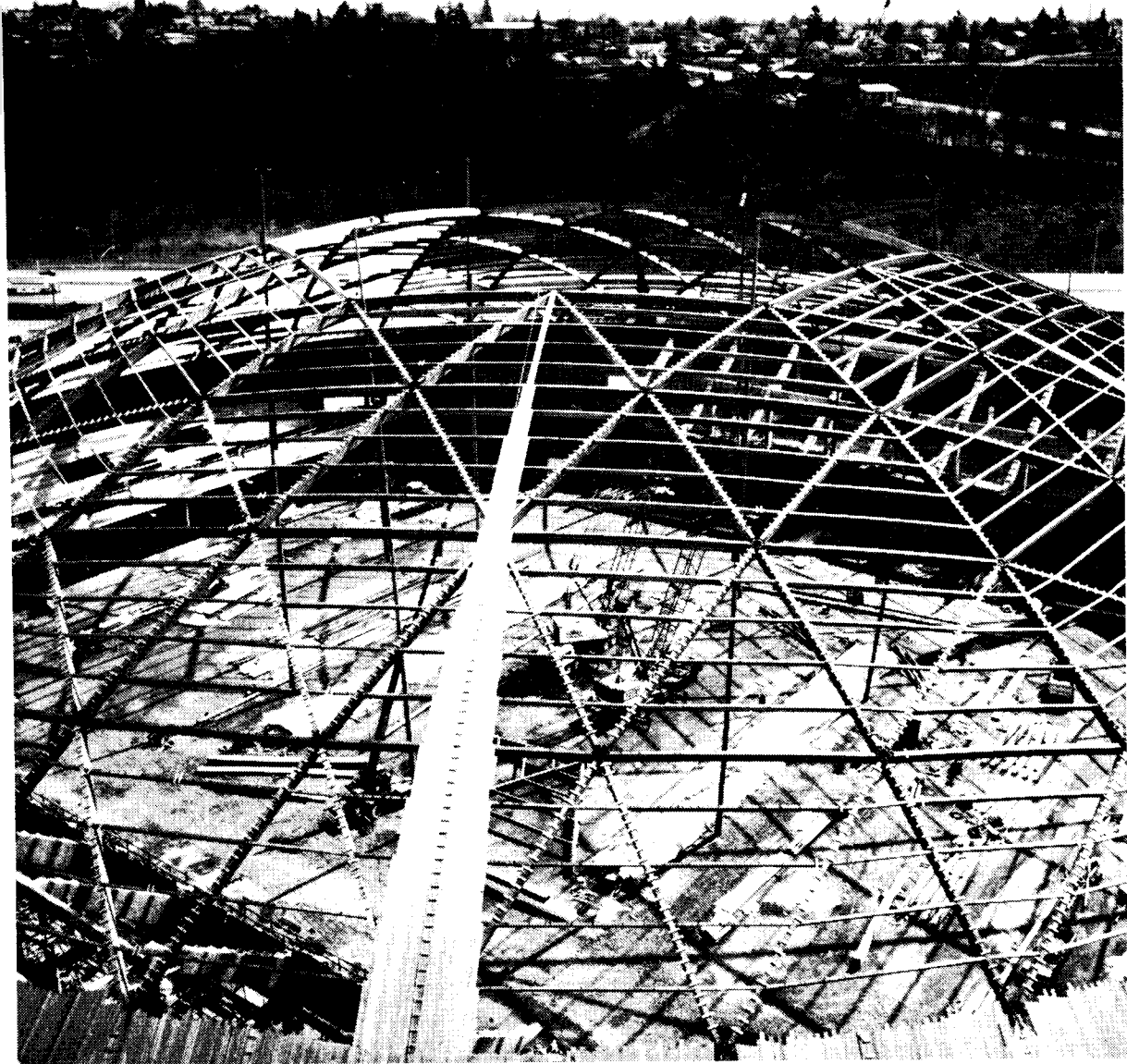
Figure 5-9 An overhead view of the Tacoma sports dome whose structure, including all long ceiling beams, is entirely of wood. The beams are made of dielectrically bonded laminated wood.
