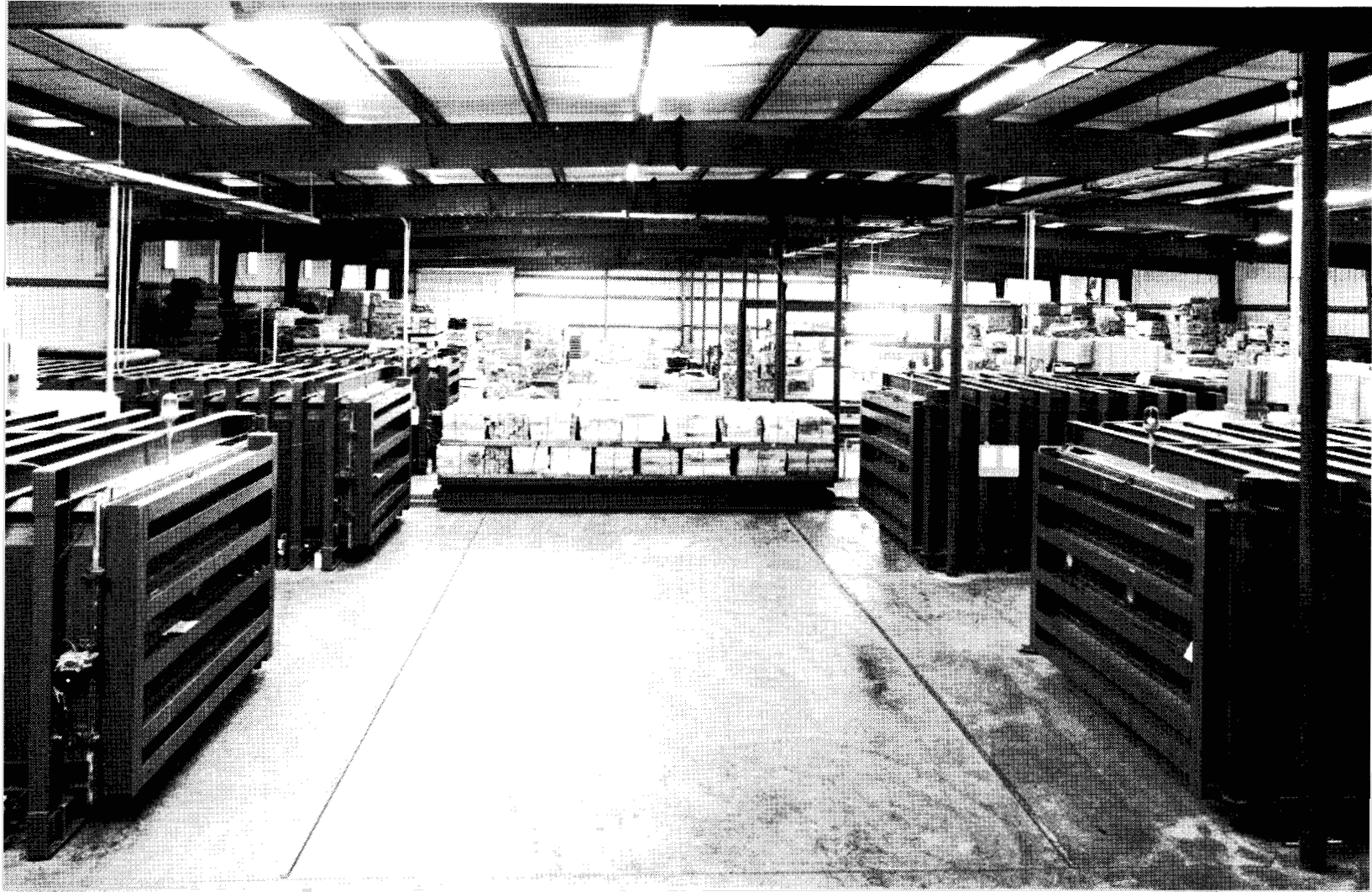
Figure 5-21 Five Lumber Drying Chambers are Shown With a Typical Load of Lumber Ready for One Machine. The 200 KW Generators are Hidden Between Adjacent Chambers. Photo courtesy of Dimension Drying, Inc.
