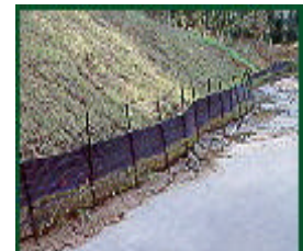
An example of a BMP: silt fencing
