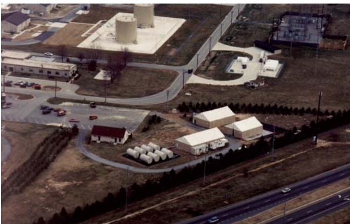
Aerial View of the DNTS showing support building, waste tank farm, and Rubb structures enclosing contained-release test cells.
