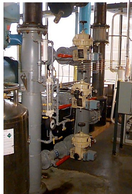
Figure 3: Primary Regulator Valves
