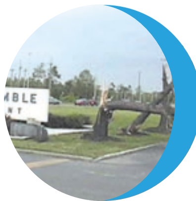
A tornado struck P&G's Pringles plant in Jackson, Tennessee, last spring.
