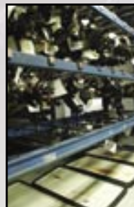
Place drip trays under stored components that may leak oil
