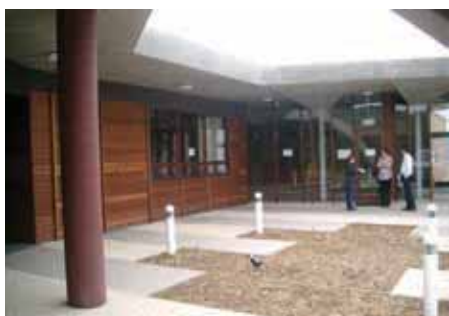
Figure 12. Queenscliff Ecocentre - courtyard, DPI Victoria.
