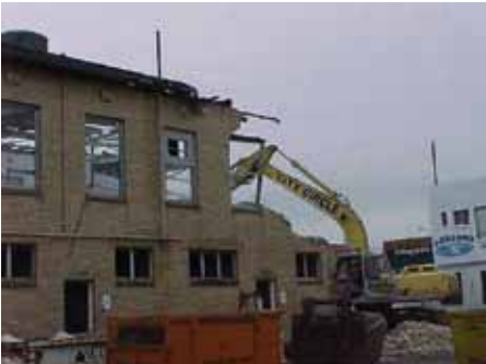
Figure 34: Old building demolition for reuse, Reservoir Civic Centre, Darebin City Council.
