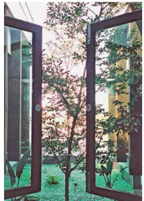
Figure 32. Roof garden with use of recycled glass mulch, Reservoir Civic Centre, Darebin City Council.
