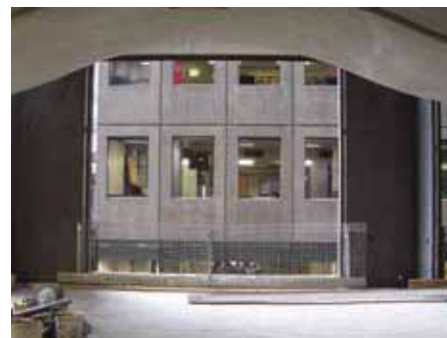
Figure 8. CH 2 construction image, vaulted ceilings from inside looking out, City of Melbourne. (6 Star, Green Star - Office Design v1)
