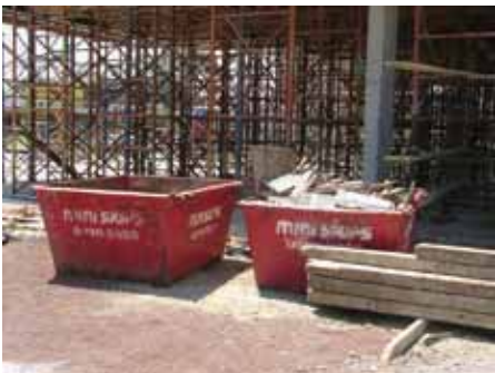
Figure 35: Old building demolition for reuse, Reservoir Civic Centre, Darebin City Council.
