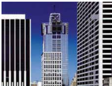
Figure 23. Photovoltaic curtain wall, image sourced from Doncaster Hill Sustainability Guidelines , Manningham City Council.
