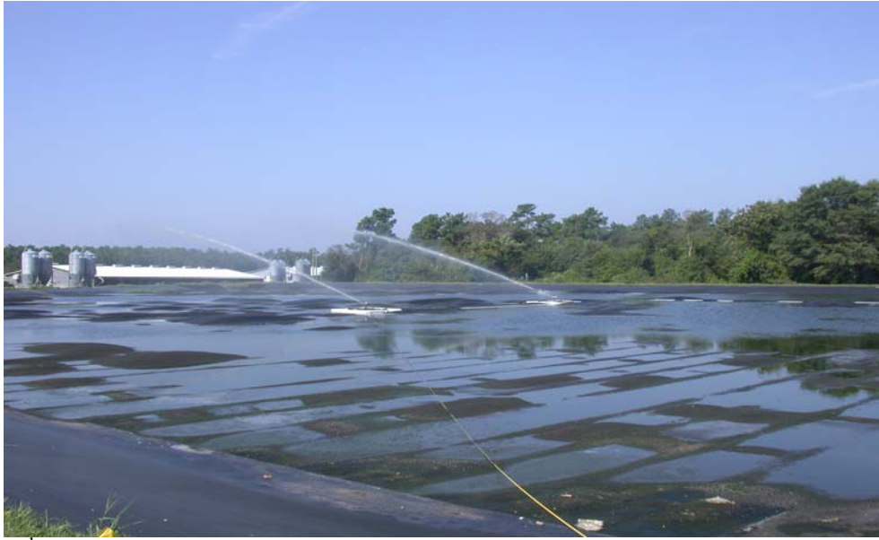
3 rd Evaluation: Irrigation at the permeable cover
