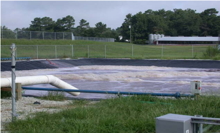
1 st Evaluation: view of aerobic digester
