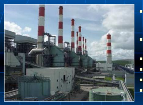
Limestone wet scrubbing systems have been installed for the power generating stations unit 4 to unit 13 The efficiency of SO<sub>2</sub> demolition are approximately 92 – 97% SO2 produced = 0.68 [Mton/year] Limestone consumption = 1.20 [Mton/year] SO2 Emission = 0.03 [Mton/year] Byproduct Gypsum = 1.92 [Mton/year]
