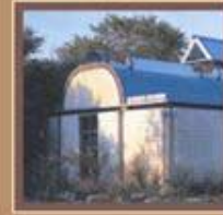
Advanced Green Builder Demonstration, Austin, TX
