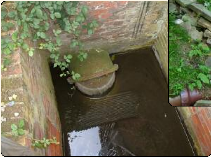
The photo above shows decaying 20th-century water supply pipe. To the left, a water sump for a 19th-century wind-powered system is shown.
