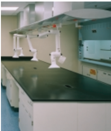
Overhead snorkels and VAV fume hood.
