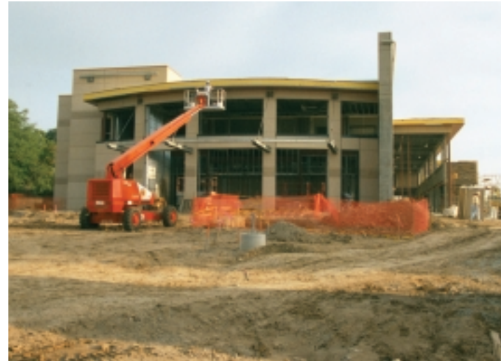
Main entrance under construction.
