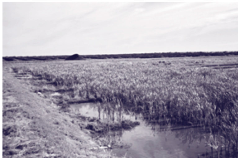
Wetlands can be used to collect and treat contaminated runoff from livestock operations.
