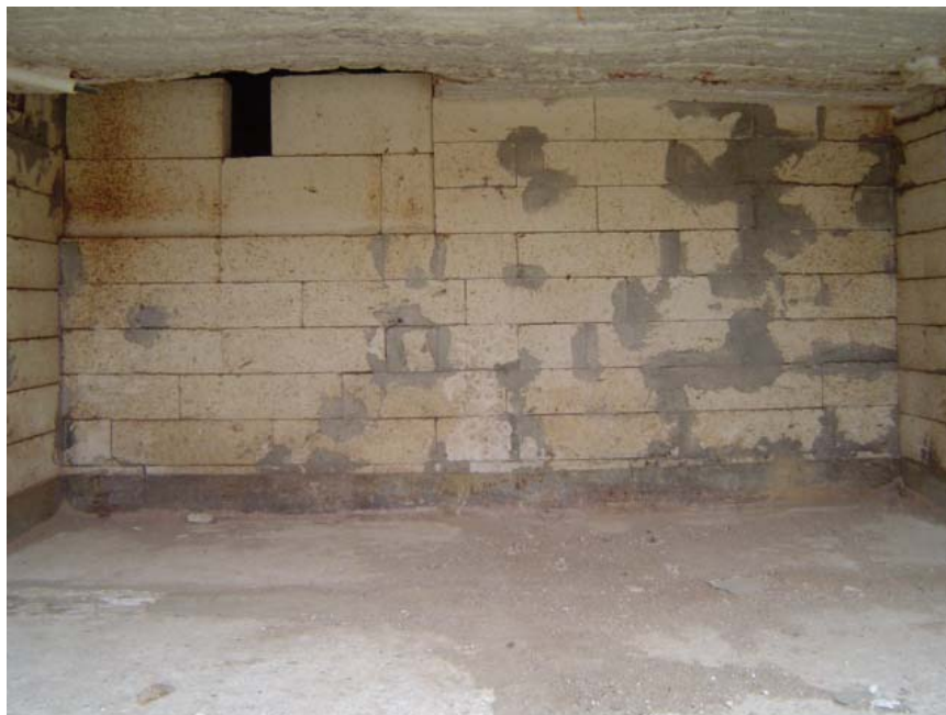
Figure 2. View of the primary chamber interior. The opening in the back drafts product gases into the secondary chamber and burner flame.
