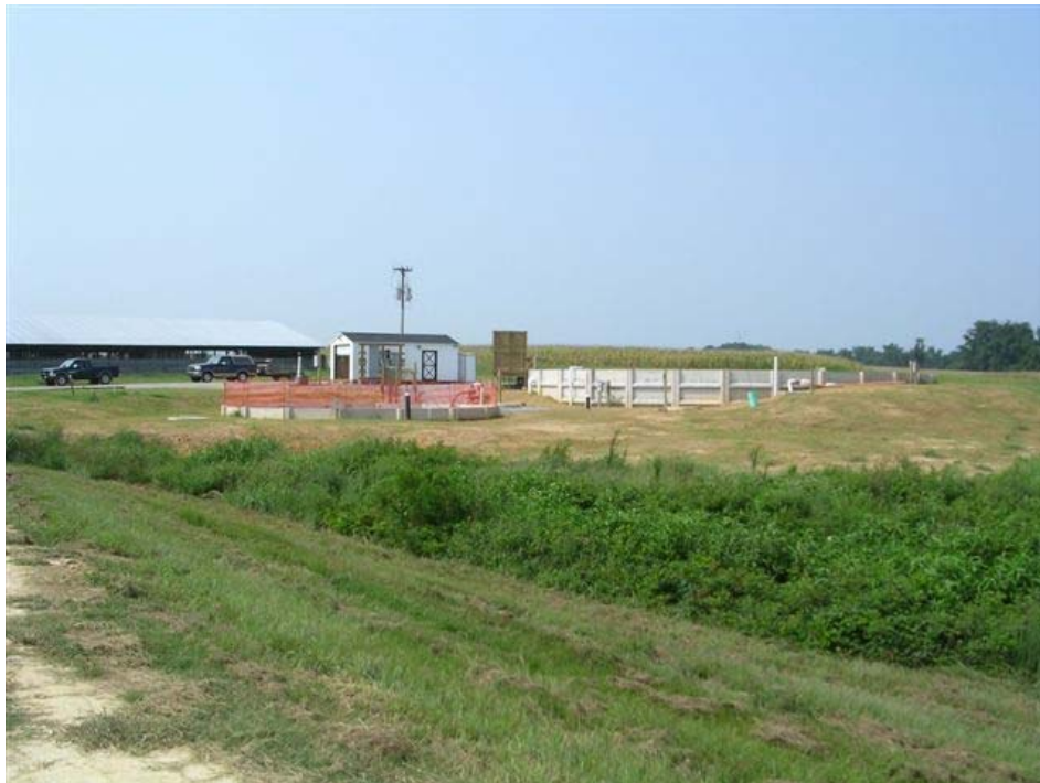
SBR system under construction
