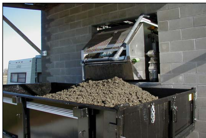
Figure 5: Separated solids from the on-farm wastewater treatment system at Goshen Ridge farm.
