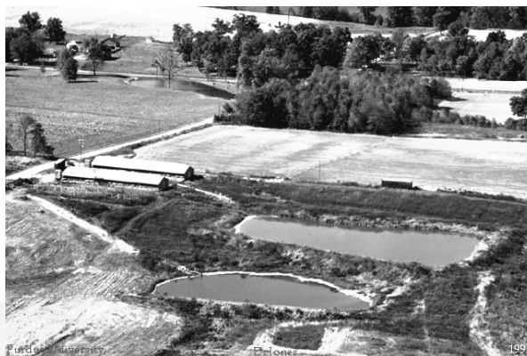
Figure 1. Two-cell manure lagoon
