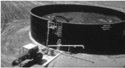
Figure 2. Fabricated steel manure storage
