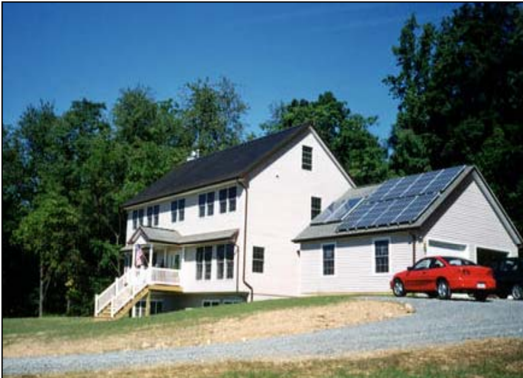
Figure C3. The Solar Patriot house at its permanent location in Purcellville, Virginia. (Photo by Ed Hancock)
