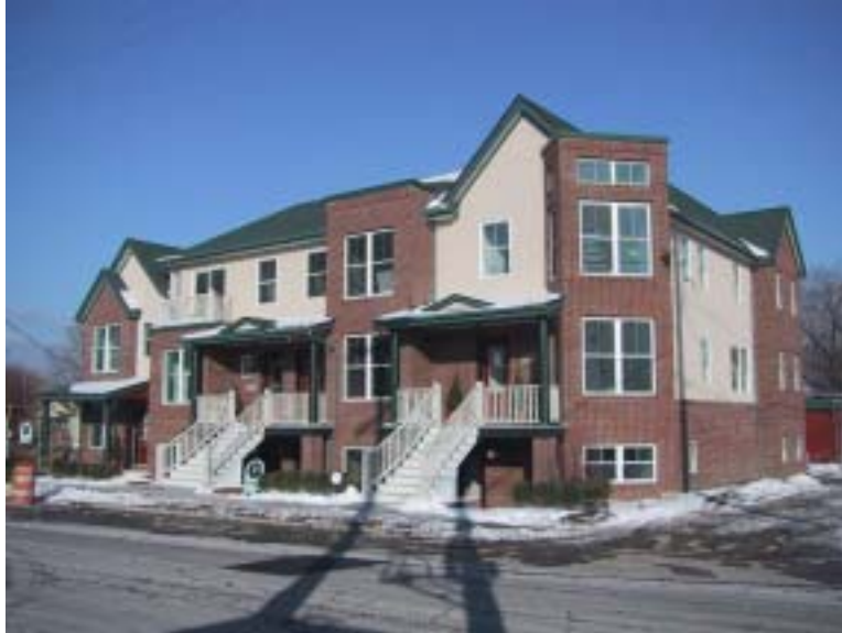
Figure C1. EcoVillage Building A (Cleveland, Ohio, December 2002)
