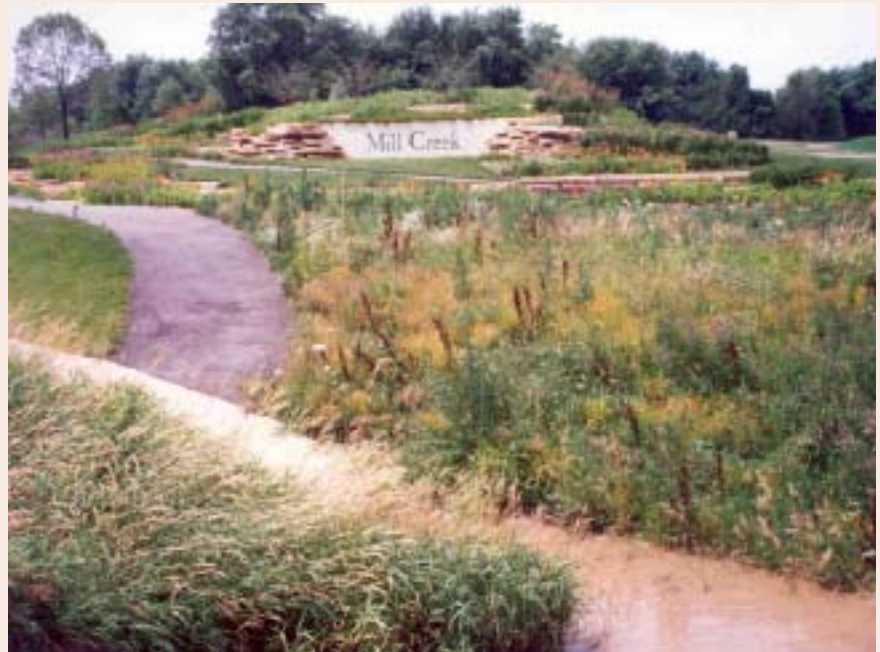
The Sheaffer System at the Mill Creek development in Glen Ellyn, IL, (1,689 homes, 133 town houses, school, and golf course) includes components such as nonstructural drainage systems (above) and stormwater detention basins (below). Photos courtesy of Sheaffer International.
