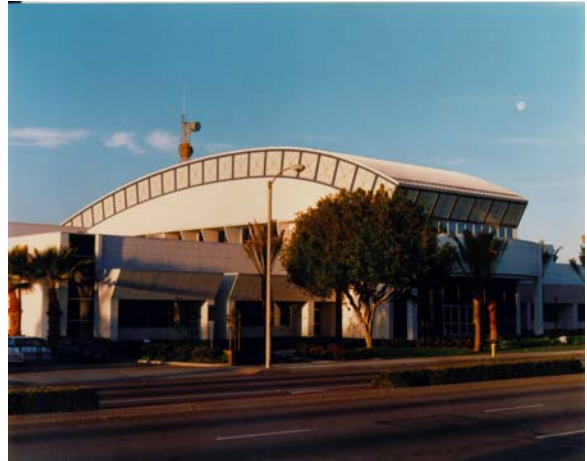
The Energy Resource Center in Downey, Calif.
