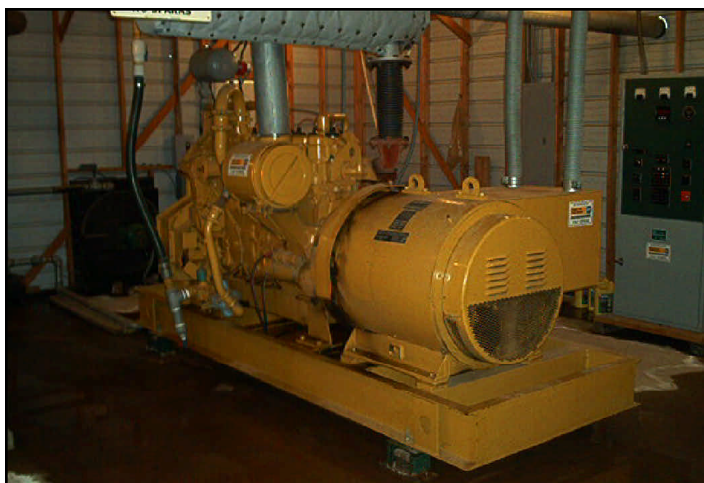
Figure 1. Engine/Generator Set Operating on Biogas from Swine Waste at Barham Farms (courtesy Julian Barham, Dr. Alex Hobbs)
