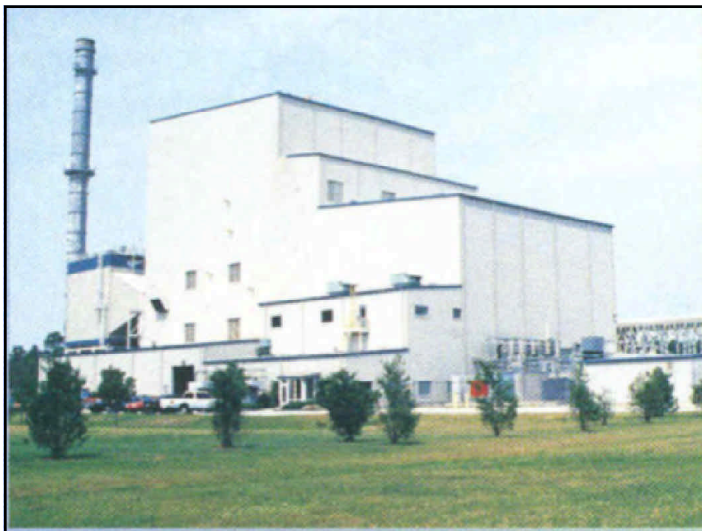
Figure 5. Craven County Wood Energy Plant (courtesy Wade Bennett)
