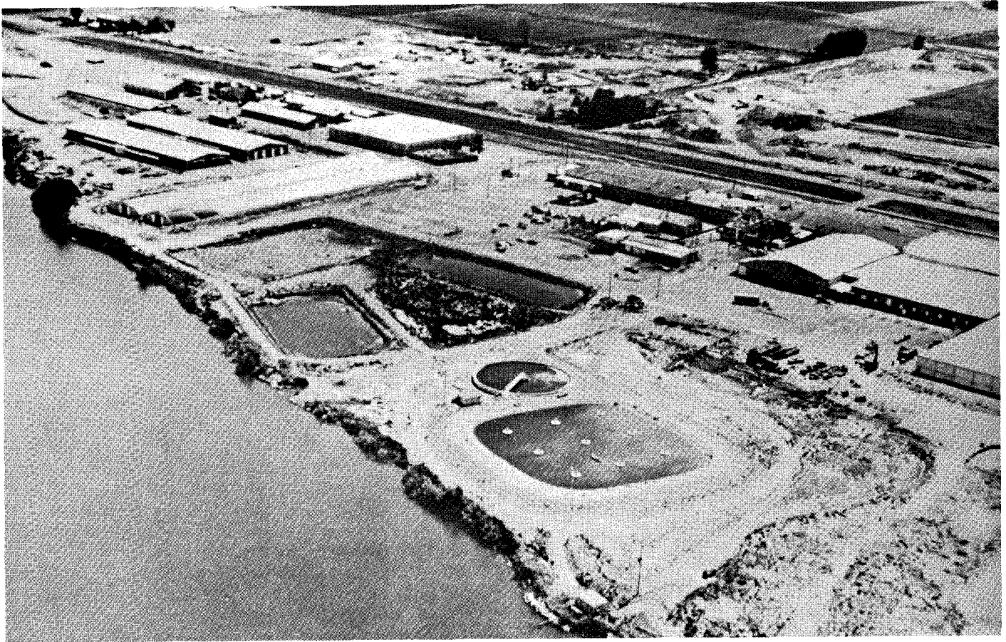
Figure 4.15. Activated sludge plant.
