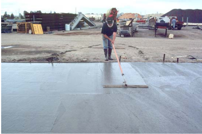
Fig 17. Finishing of cullet concrete
