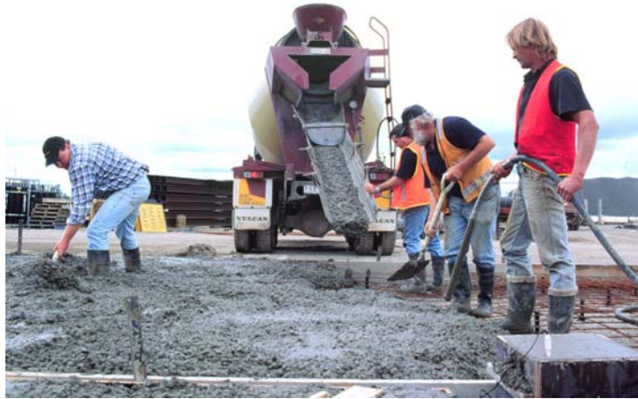
Fig 15. Placement of cullet concrete
