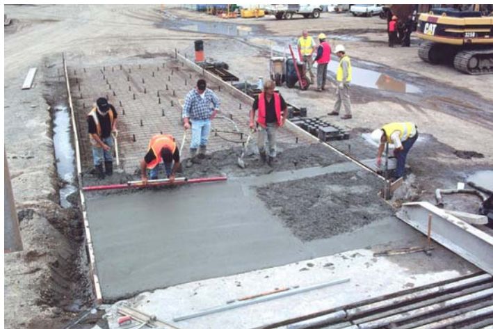
Fig 16. Finishing of section of glass cullet concrete
