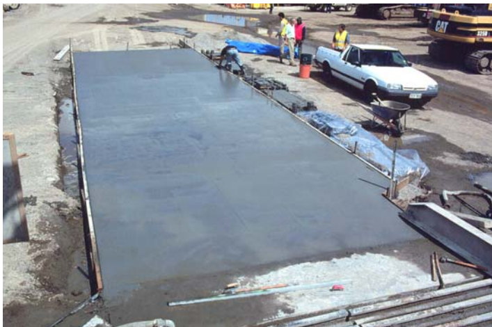
Fig 18. Finished cullet concrete for curing
