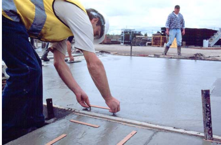
Fig 19. Instrumentation of cullet concrete to monitor concrete dimensional stability.
