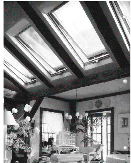
Figure 21: Operable skylights provide daylighting and natural ventilation.
