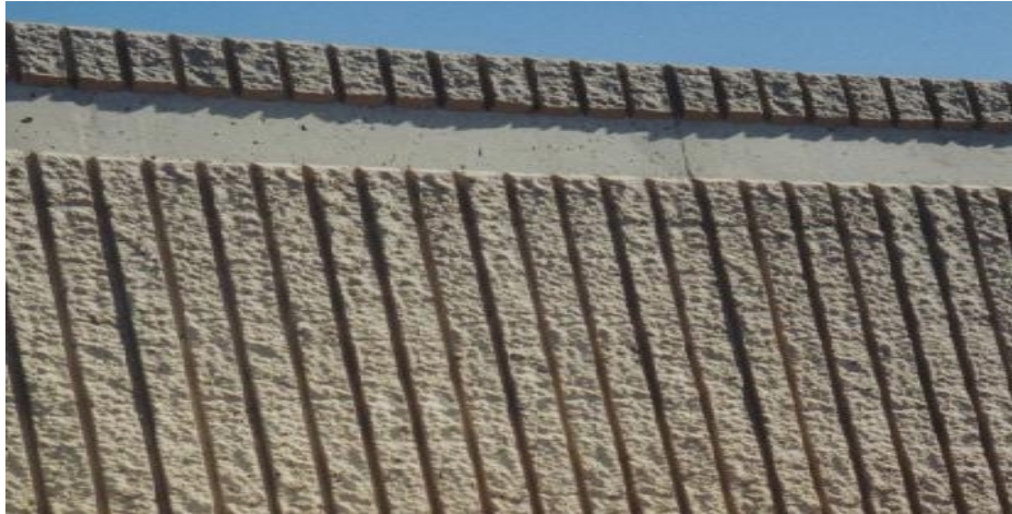
Figure-1 Grooved noise barrier walls near Highway 101 in Tempe, Arizona
