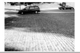
**Description**: Modular block porous pavement is a permeable pavement surface with an underlying stone reservoir designed to temporarily store surface runoff before it infiltrates into the subsoil. Porous pavement options are primarily intended for low vehicle traffic areas such as spillover parking or simply the parking aisle portion of a parking lot.
