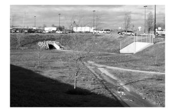
**Description**: Dry extended detention ponds (a.k.a. dry ponds, extended detention basins, detention ponds, extended detention ponds) are basins designed to temporarily detain runoff for some minimum time. Dry detention ponds are used for water quantity control only, and can also be used to provide flood control by including additional flood detention storage.
