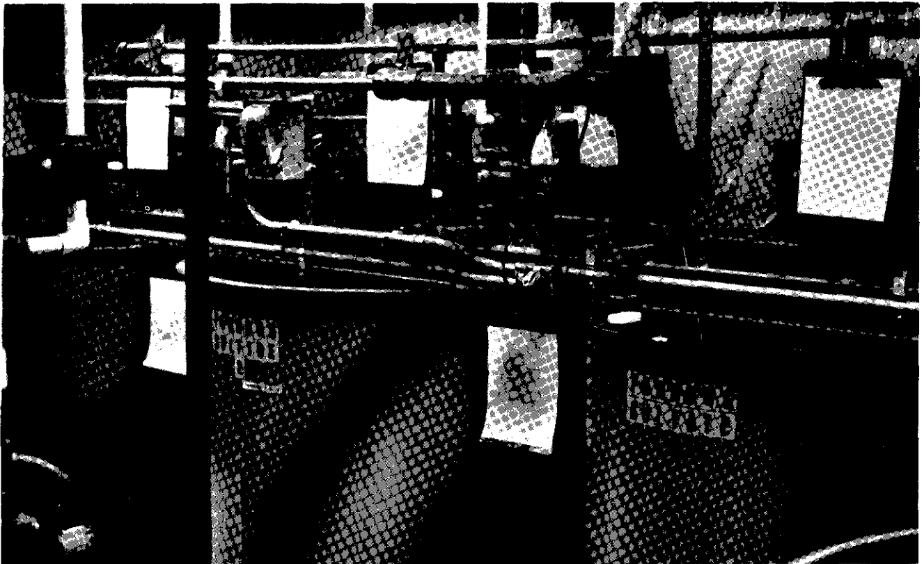
Ferrous sulfide makeup and feed system
