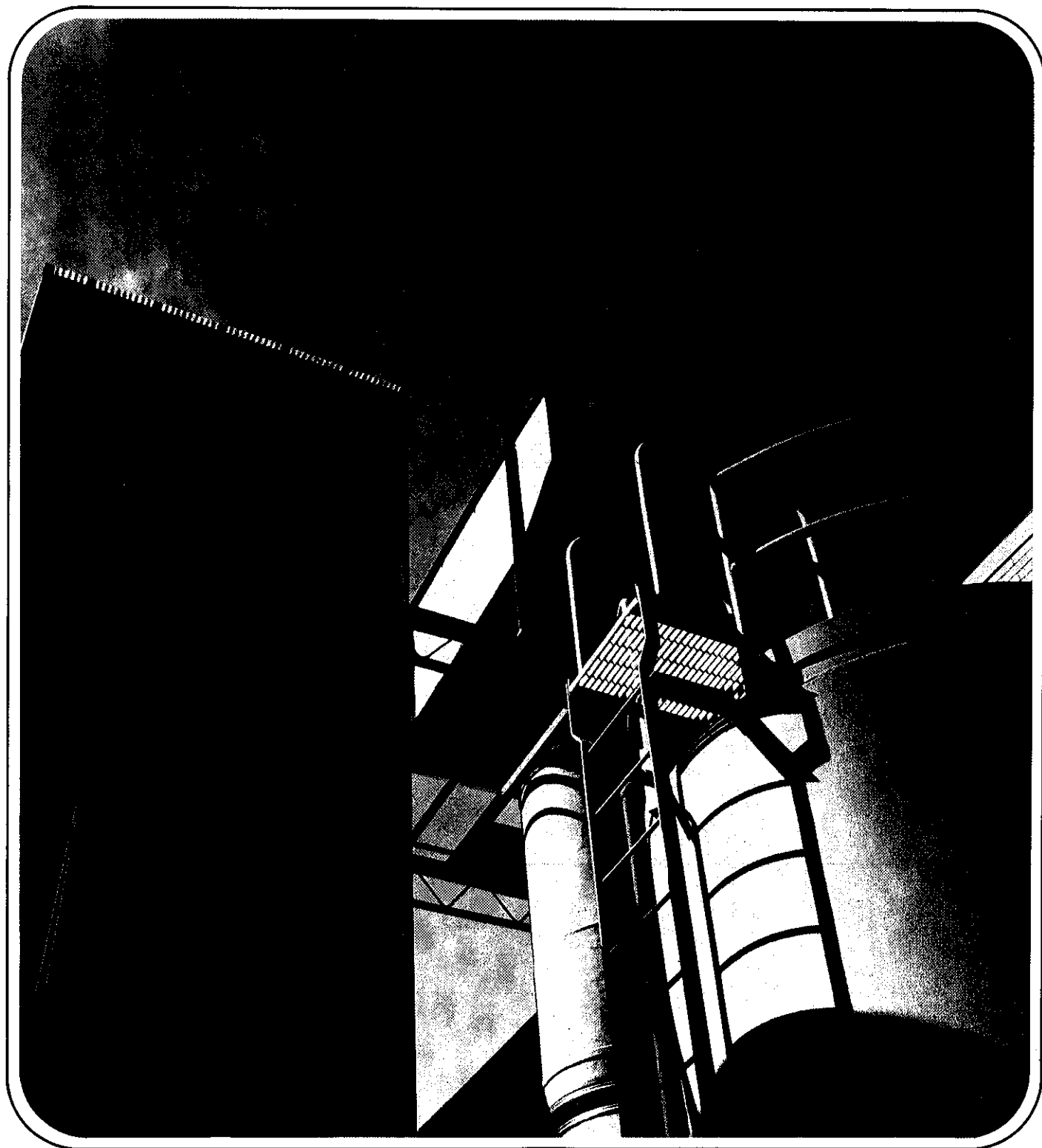
Acid recovery tower (left), acid mist filter (center), fresh acid storage tank (right)
