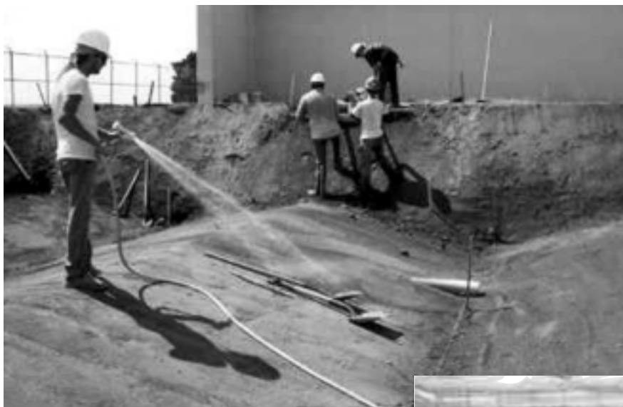
The Mars company's reed bed at Waco, Texas, under construction: (left) shaping the sand and (below) pulling the liner into position.
