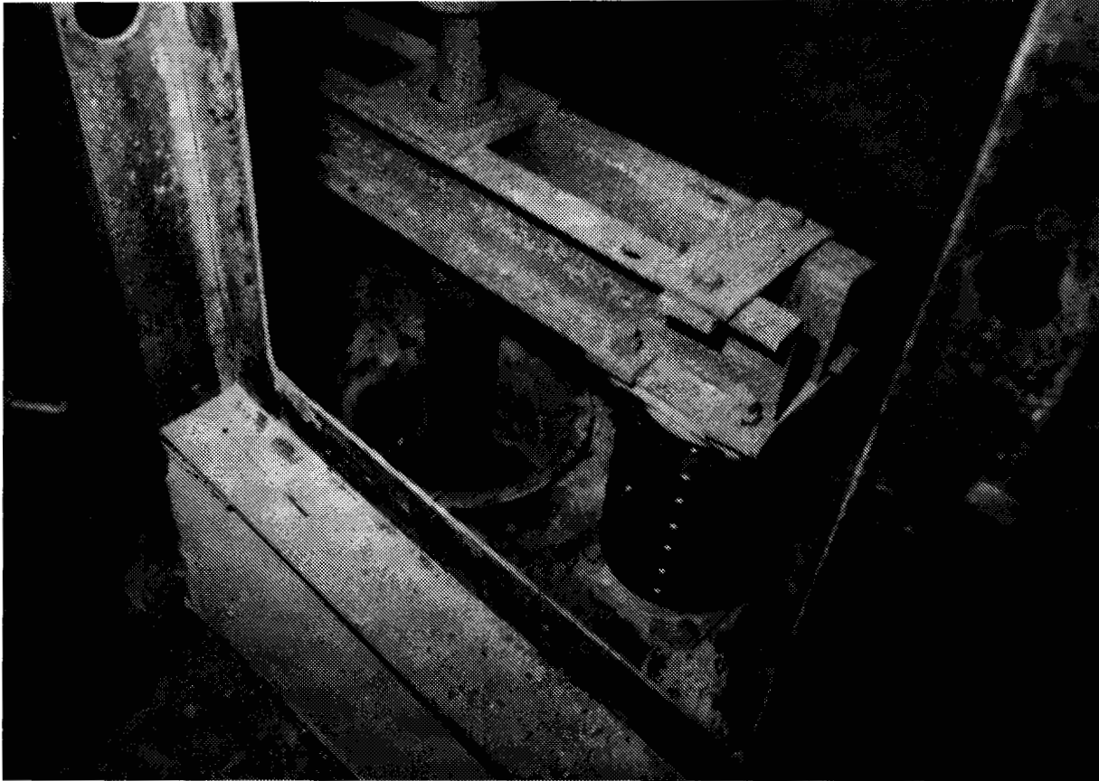
Figure 6-18. Access to a typical insulator enclosure and support insulator for the discharge wire frame.
