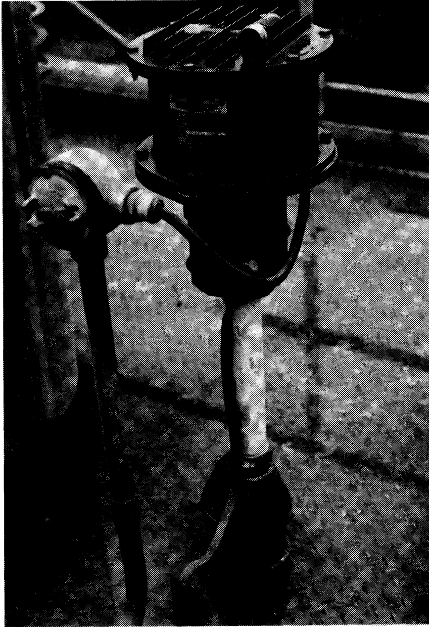
Figure 2-20. Typical electric vibrator type rapper.
