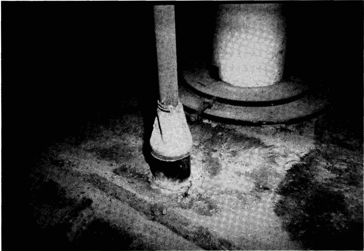
Figure 6-28. Jack screws.
