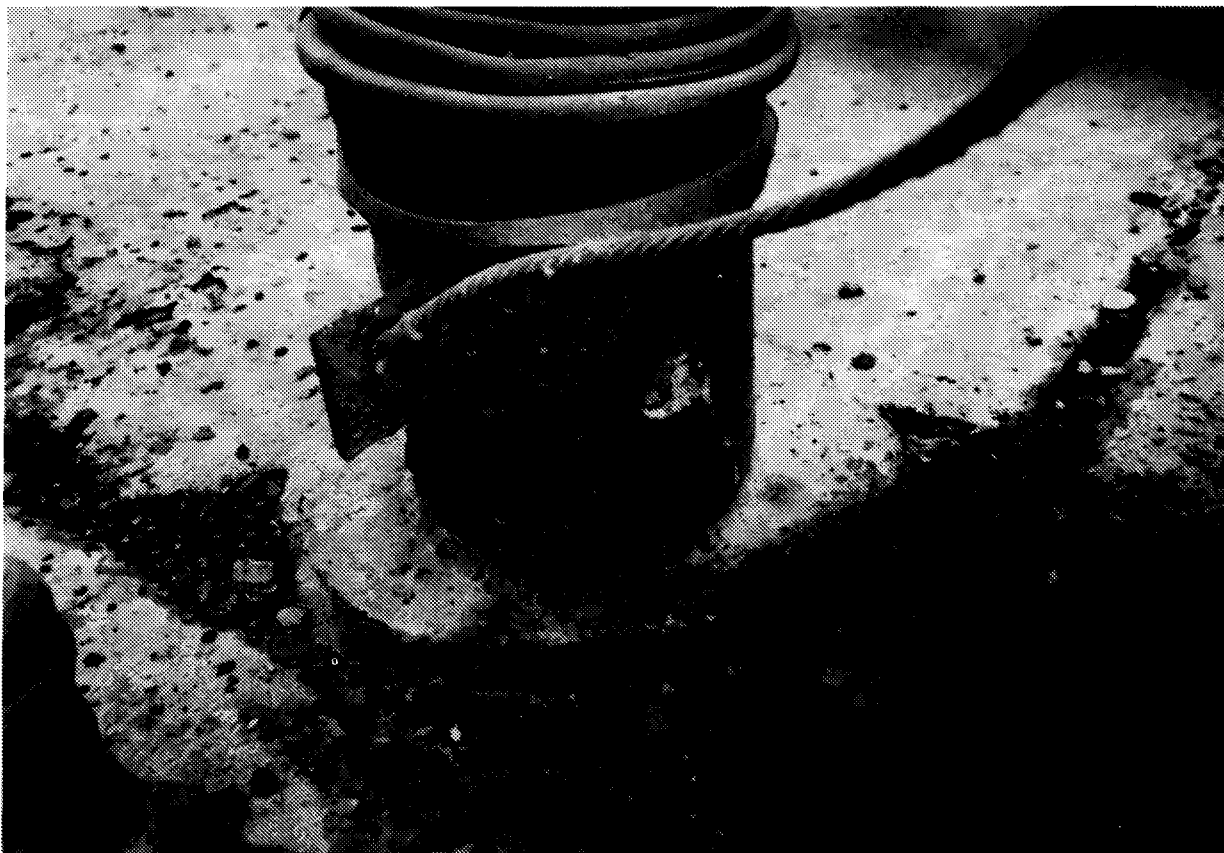
Figure 6-4. Example of rafter boot corrosion.
