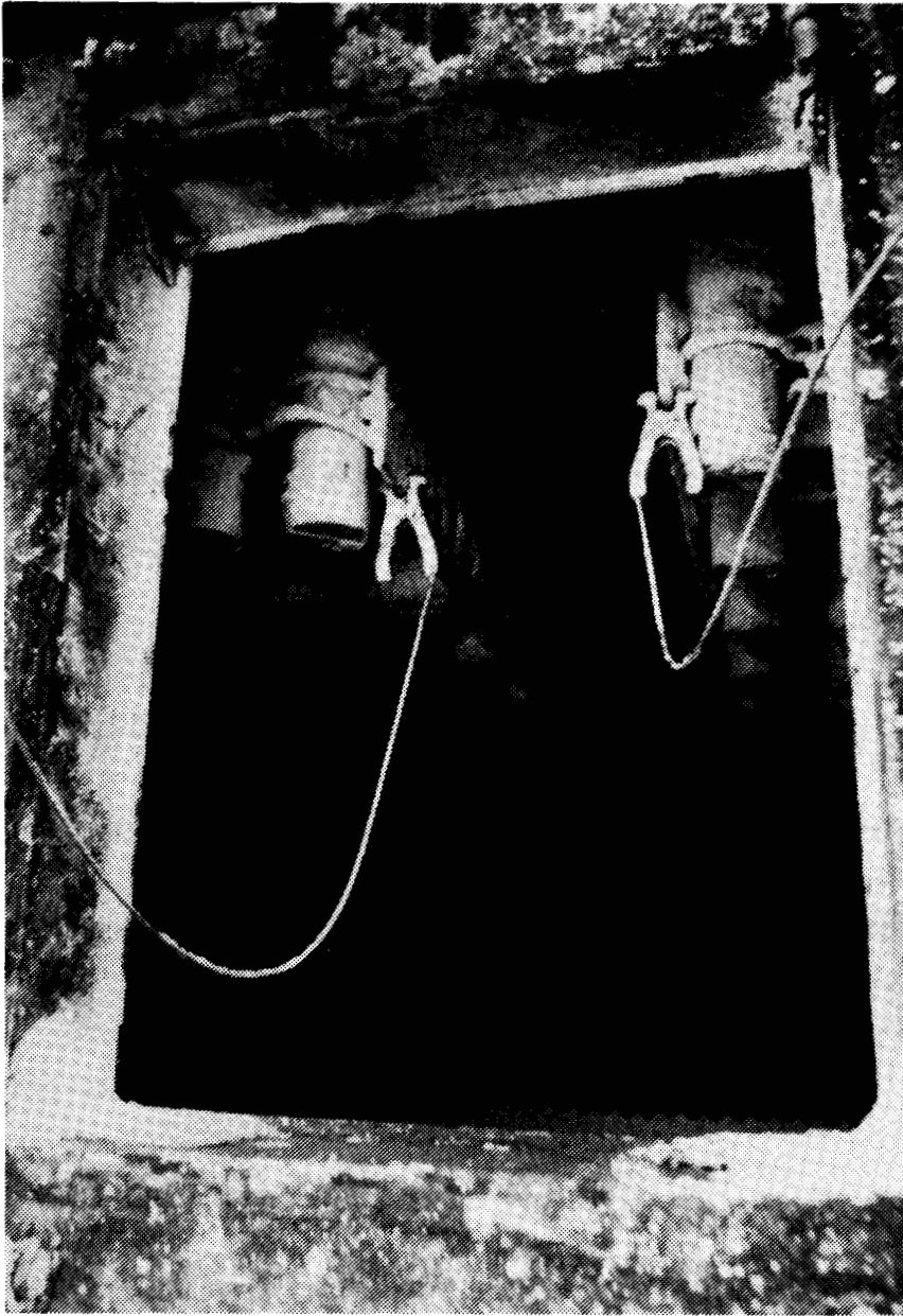
Figure 7-3. Ground clips.
