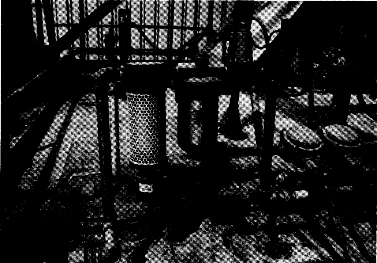
Figure 6-1. Rapper air line trap and filter.
