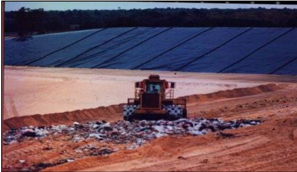
Landfill liners (background) are required in all Class I and II landfills in Florida.
