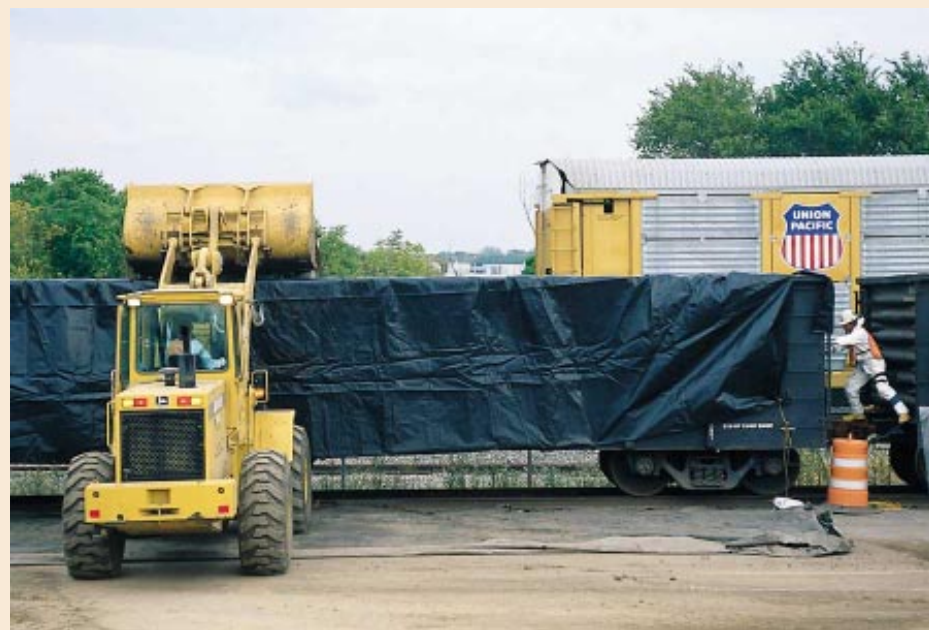
Rail cars are used at a FUSRAP site to transport contaminated soil to a processing facility instead of trucks because it is more efficient and cost-effective.
