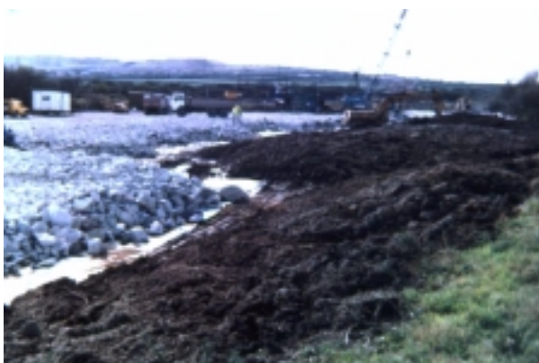
Embankment constructed using china clay waste
