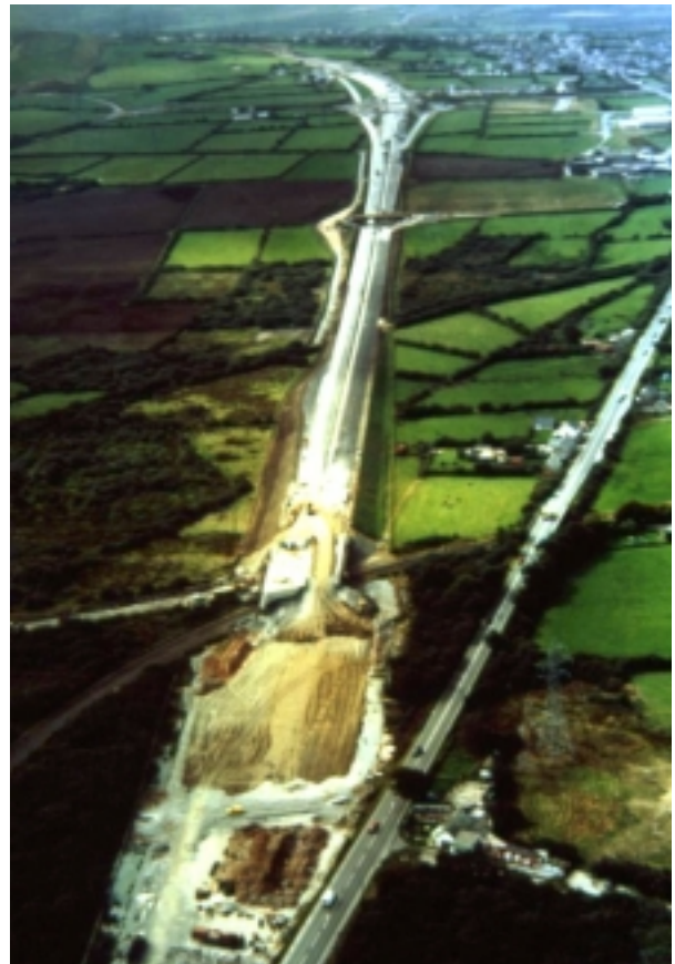
A30/A39 Indian Queens and Fraddon Bypass during construction
