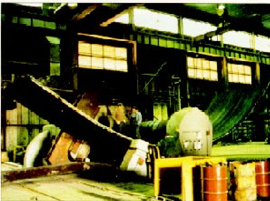
Sparks fly as a worker grinds the edges of a service opening (top). A steel plate 3 inches is bent to form a section of one of the three steel rings that were welded together to the pressure vessel shell (bottom). Prefabricated at B&W's facility in Mt. Vernon, Indiana, the pressure vessel stands ready for removal of the top head and installation of internal components (opposite).
