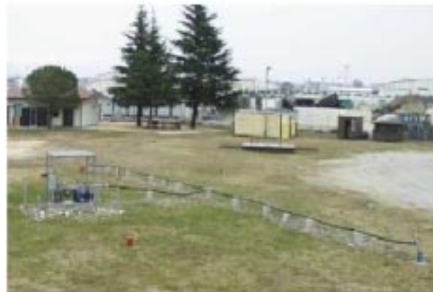
North POL Facility
